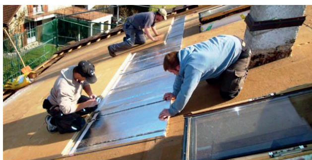
Pose des plaques isolantes Vakutherm.
