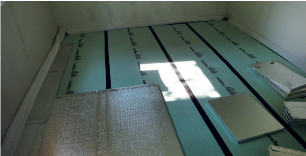
Coller proprement les raccords.
